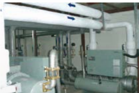
Machine Room for Conventional Central Water-source Unit
